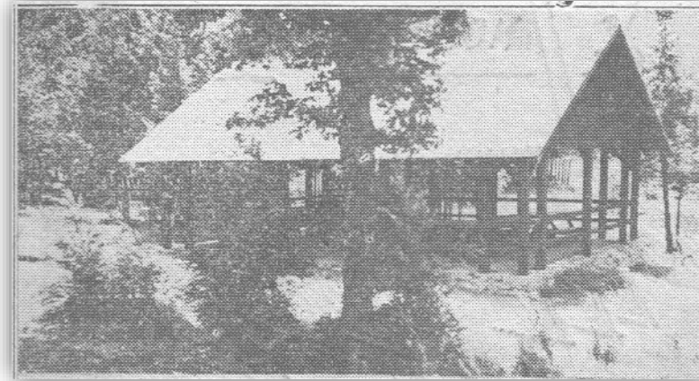
The pavilion built by CCC workers at Bucks Creek Area Park. Today only the steps and foundation are visible.
