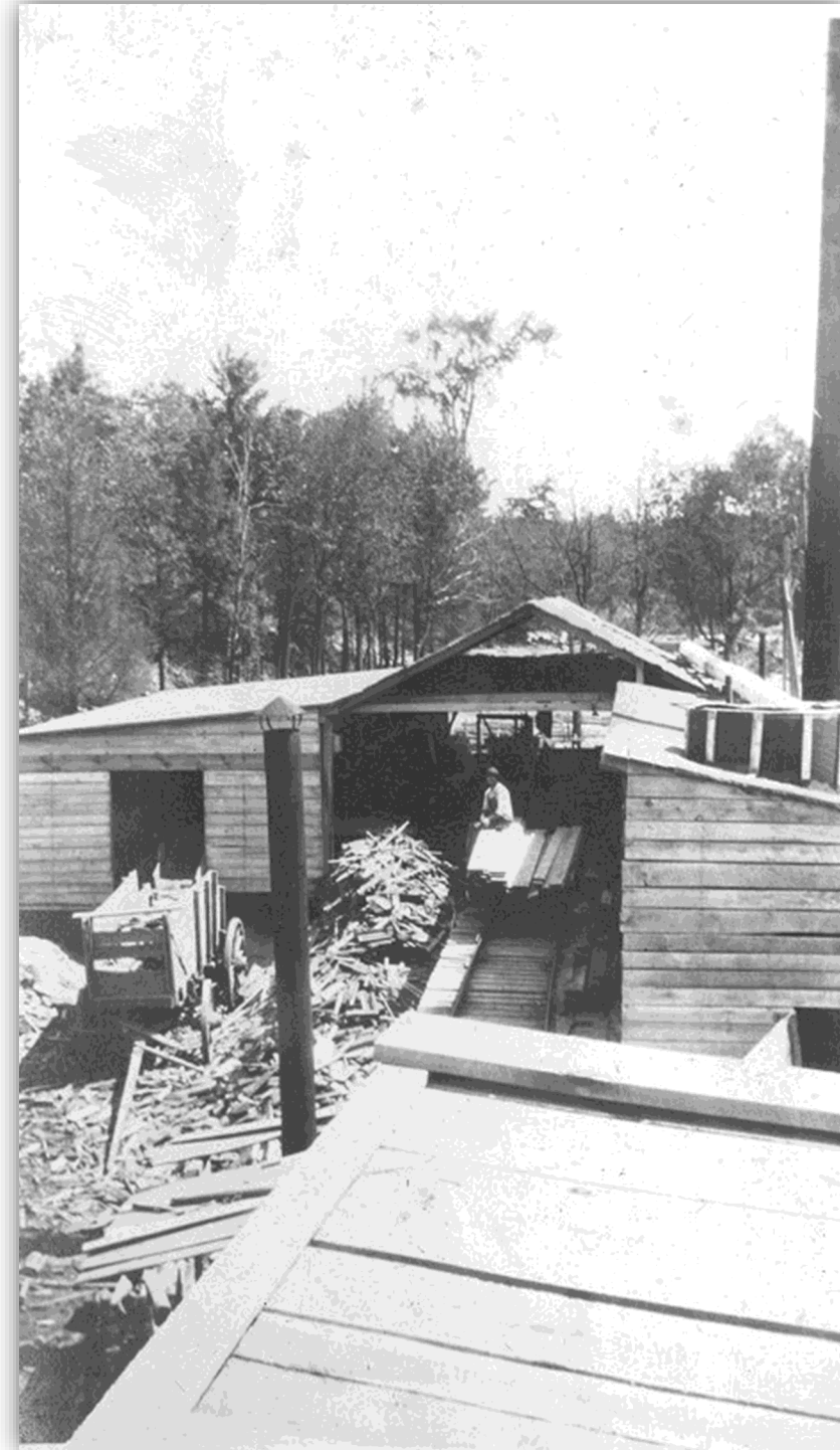
Photo probable circa 1910-20. Oral histories record this as Braman's Mill located within a mile of Woods Mills, NY. This sawmill in photographs does not appear to be water powered but looks like it may have used steam or coal to power it. No archaeological remains of this mill have been found.
