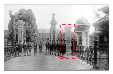
Building 2310, known as the White House has Japanese constructed arch stone bridge and stone gateposts. The stone bridge is used only for pedestrian traffic. The bridge and gateposts remain in good condition. The right photo shows Japanese army guards standing at the gate. Metal bars protruding from the post that originally held the iron gate are still visible.
