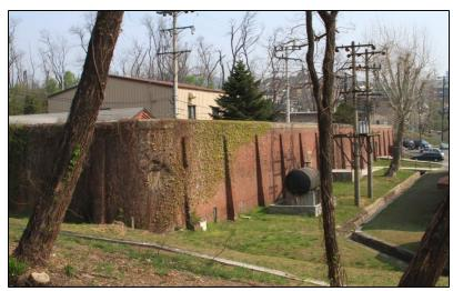
A former Japanese Stockade built in Sept 1909 after the construction of the notorious Sodaemun Prison. This stockade has a 16 ft high perimeter red brick wall. The wall is reinforced with wireframe cement. Bullet holes and damage to the wall are associated with actions that occurred during the Korean War. Building 4713 located within the wall was used for the management of prisoners. Both building 4701 and the perimeter wall are well preserved, close to its original condition.
