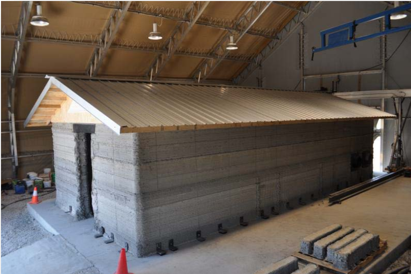
A barracks hut constructed with the Automated Construction of Expeditionary Structures is a new construction technology that prints concrete structures. The printer reduces building materials shipped by half and construction manpower requirements by 62 percent when compared to expedient plywood construction in overseas military construction. This hut resides at the Construction Engineering Research Laboratory in Champaign, Illinois. (Photo by Mike Jazdyk, ERDC PAO)
