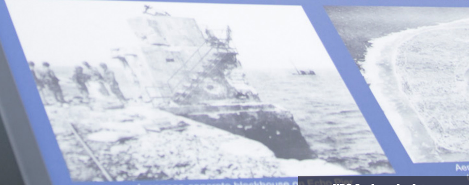
Japanese concrete blockhouse on Echo Pier
