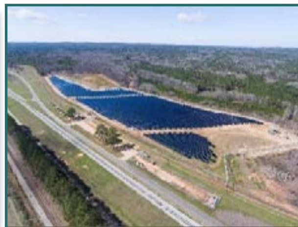
Anniston Army Depot 7 MW Large-Scale Renewable Energy Solar Project (April 2017)
