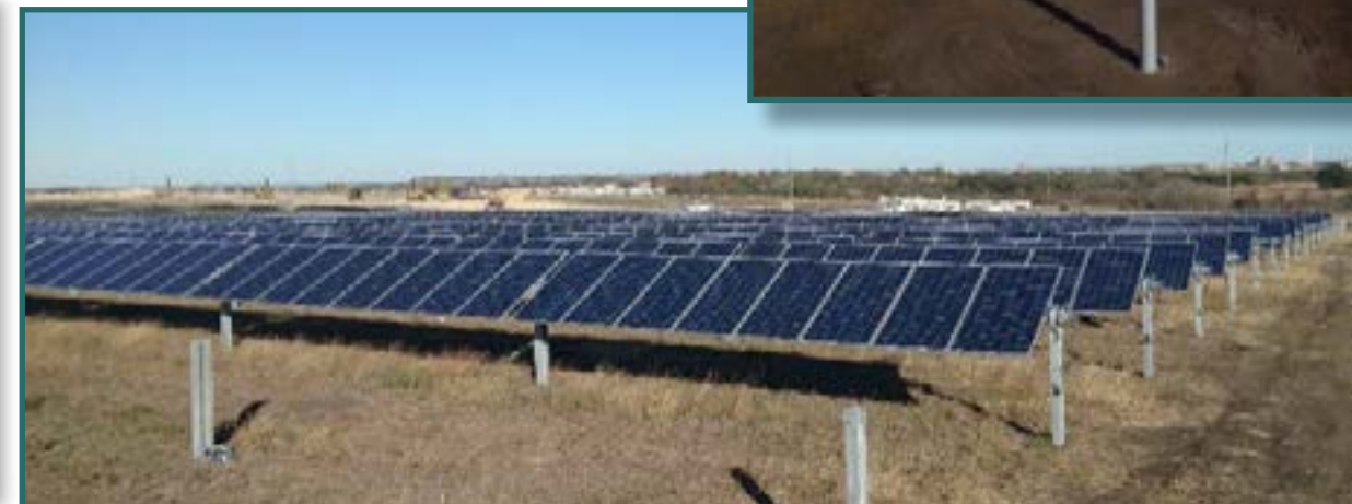
Fort Hood Large-Scale 65 MW Solar and Wind Energy Generation Project (June 2016)
