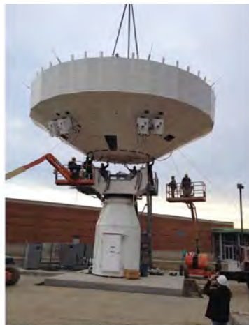
Modernization of Enterprise Terminals Installation of AN/GSC-52B(V)2 Satellite Terminal Antenna at Fort Detrick, MD
