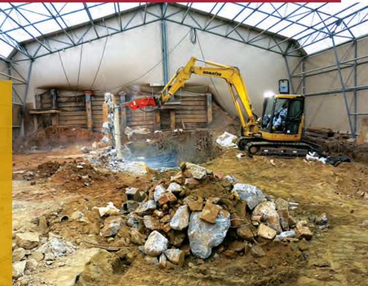
An ECBC field response team assists the Army Corps of Engineers with removal of chemical warfare material in the Washington D.C. neighborhood, Spring Valley.
