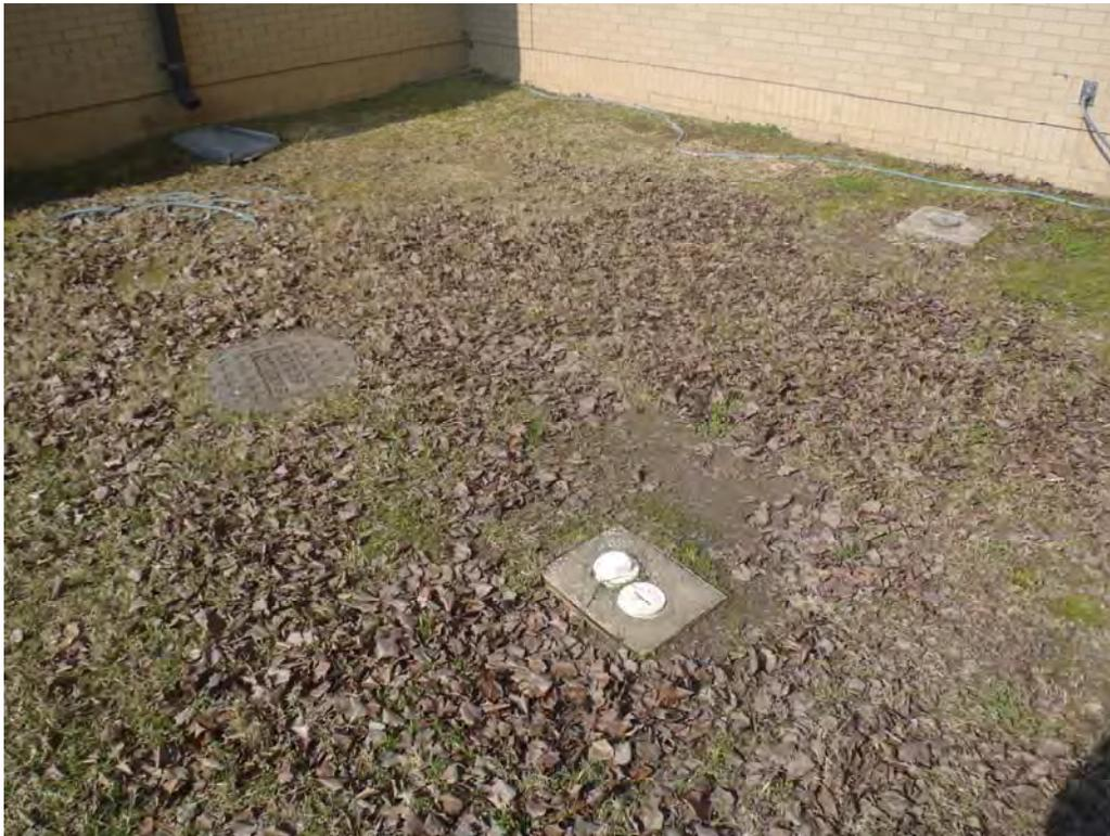
Photo 4: Grease trap cleanout facing southwest
