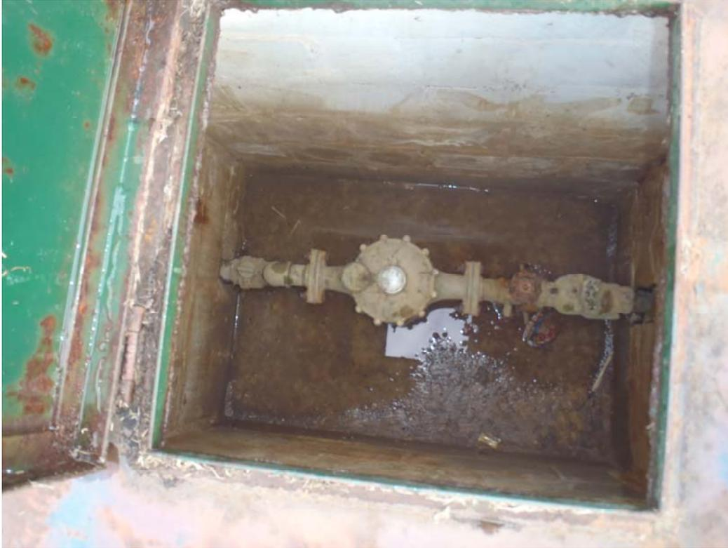
Photo 11: Water meter vault
