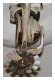
Painted sprinkler head found in a barracks room. The paint will insulate the head causing it to react up to 2 minutes slower. In less than 2 minutes, a fire can grow from 200 to 1400 degrees!
