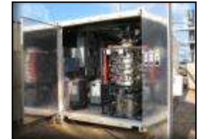
Waste -To- Energy
