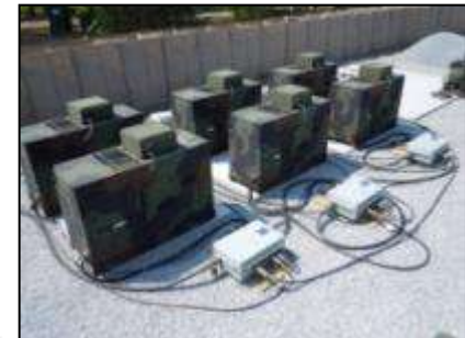
Microgrid and 60 kW TQGs
