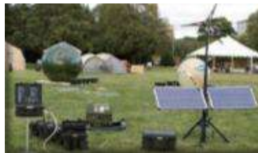
3 kW TQG w/ Solar-stik Hybrid Integrates small-scale solar & wind with batteries & Tactical Quiet Generator (TQG)
