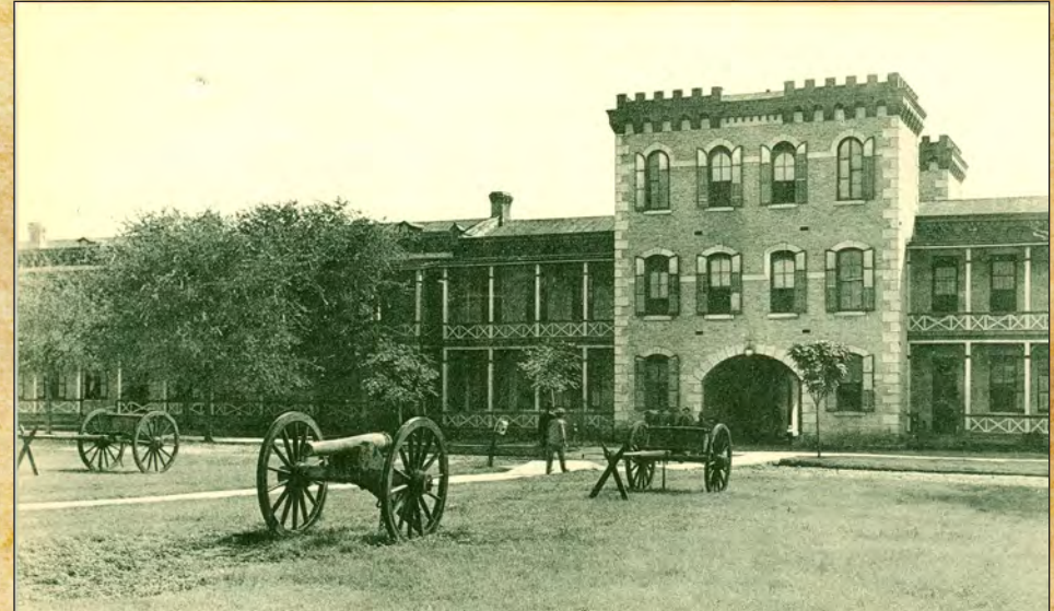
At the center of the line of barracks was Building 613 with a sally port leading from the parade ground to the service area behind the barracks.
