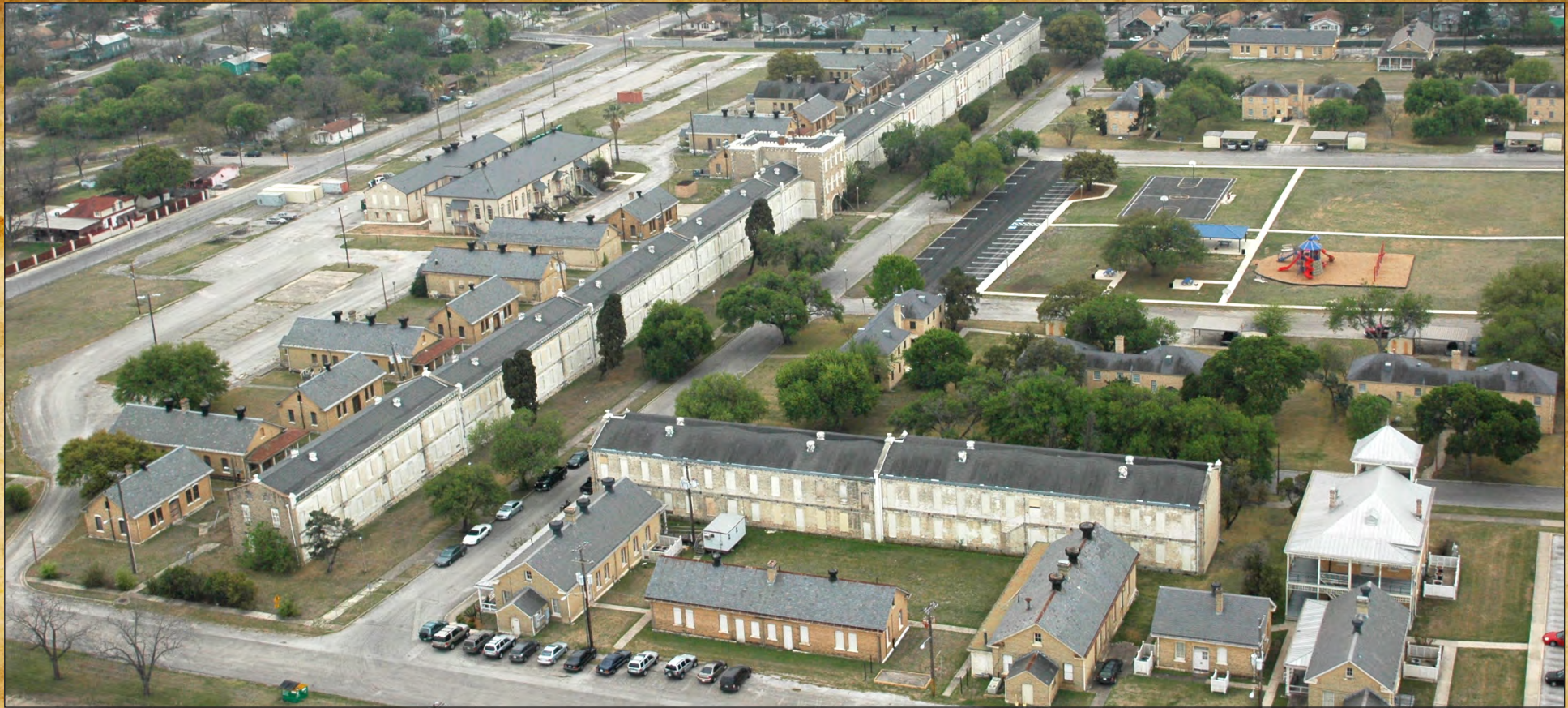
A boarded up Long Barracks in 2008 awaits renovation and new tenants following decisions made by the Base Realignment and Closure Commission.
