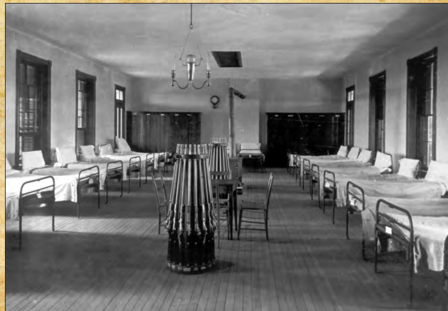
Each of the barracks had two large bays upstairs for sleeping areas for a total of about 50 enlisted men.
