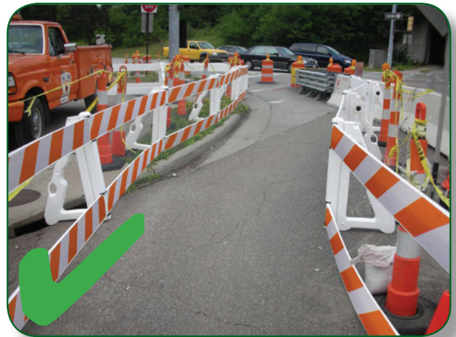
Pedestrian access should be maintained in work zones.
