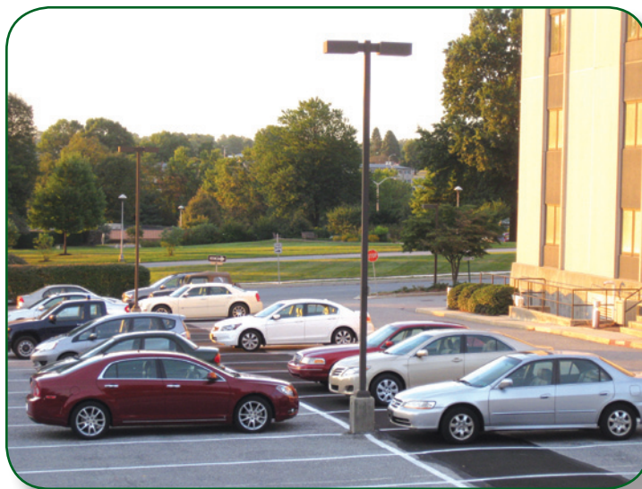
Exhibit 8. Parking Lot Lighting using Full Cutoff Lamps
