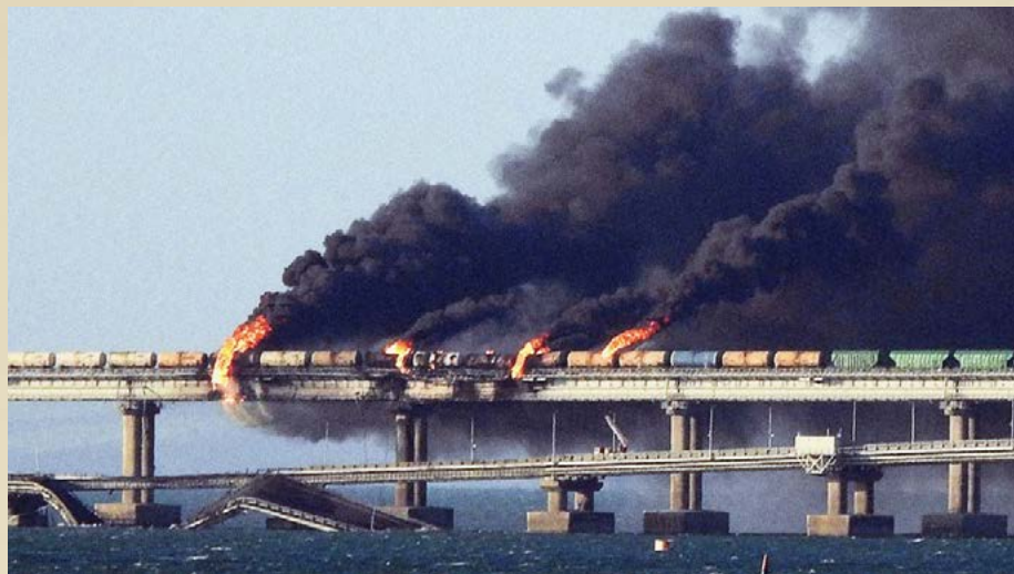
October 2022 attack on Kerch Straits Bridge
