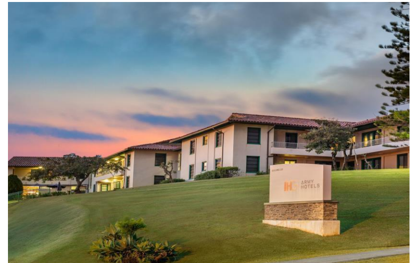
IHG Army Hotels Building 228
