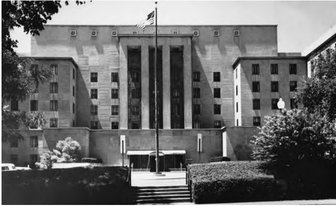
New War Department Building
