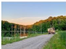
Road clearing and investigations
