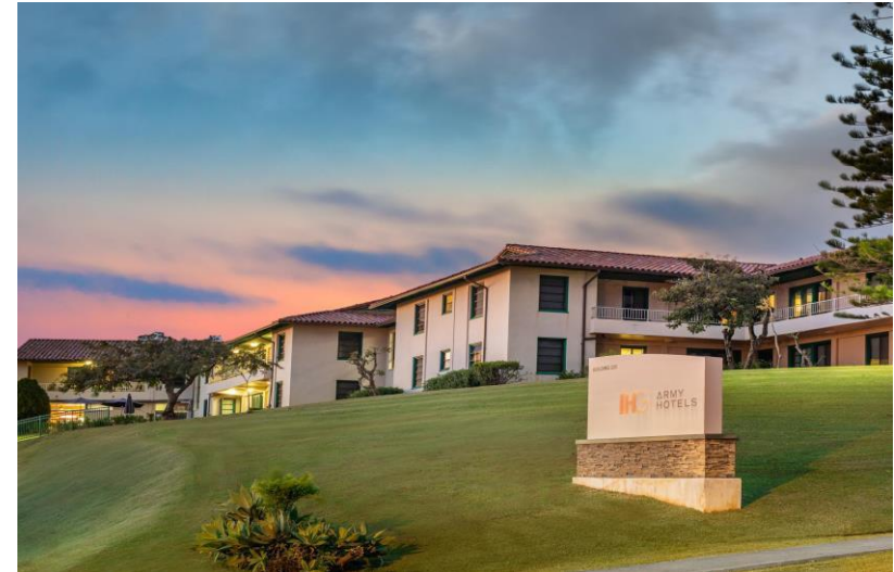
IHG Army Hotels Building 228
