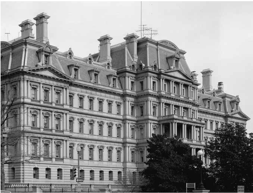
State, War, and Navy (SWAN) Building (South Façade), southeast corner of Pennsylvania Avenue and 17th Street NW, Washington, D.C., by Ronald Comedy, ca. 1933 ( Library of Congress )
