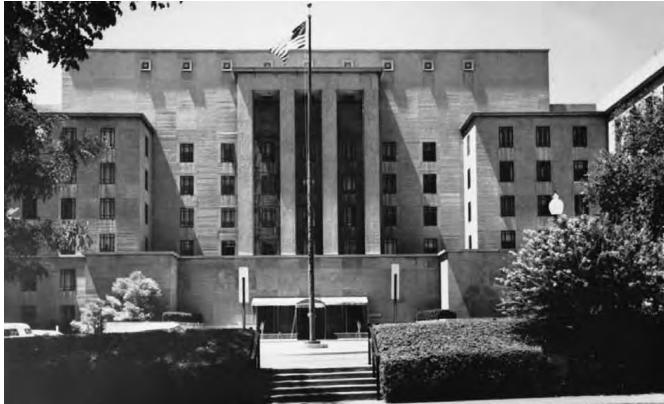
New War Department Building
