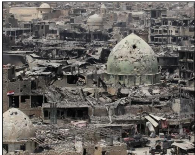
Destruction of West Mosul.
