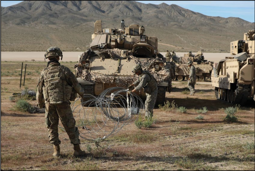
Figure 7-3. Engineers setting concertina wire
