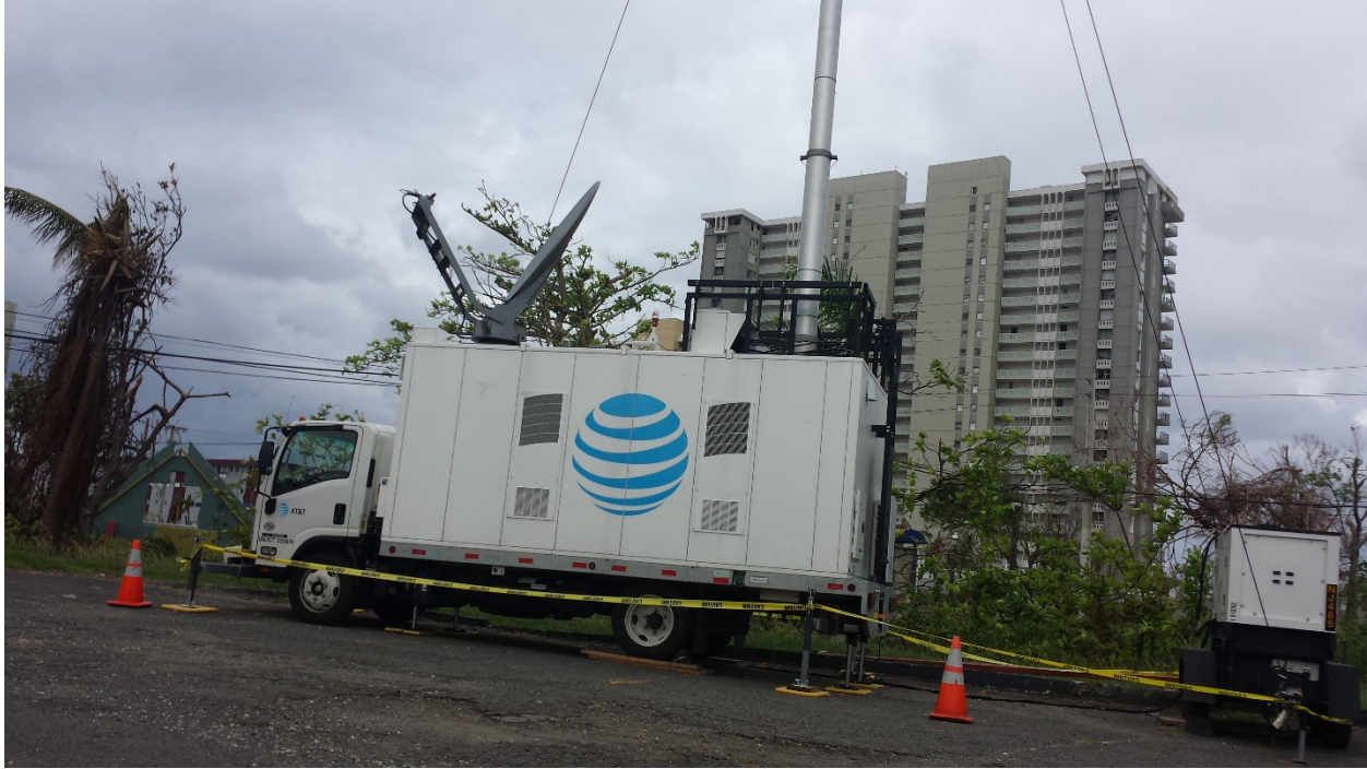
Figure 1-6 Portable mobile phone repeater van in Costa Azul, Puerto Rico
