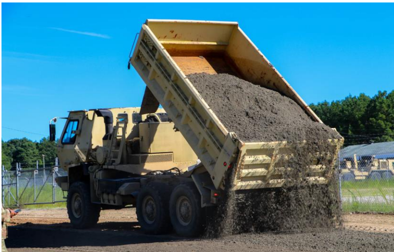
76th Engineers support Fort Pickett during AT Virginia National Guard Soldiers assigned to the Powhatan-based 180th Engineer Support Company, 276th Engineer Battalion, 329th Regional Support Group conduct road repairs and maintenance during their annual training Aug. 13, 2022, at Fort Pickett, Virginia. Using various vehicles, the engineers dropped, graded and smoothed new road surface material, which will help improve durability and safety on the repaired roads.
