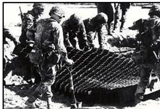
Soldiers from the 20th EN BDE repair a damaged runway (ca 1985)
