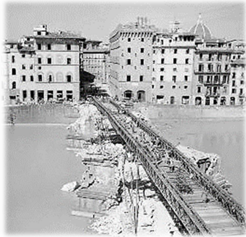
Soldiers from the 92nd EN BN (20 EN BDE) support bridging operations in Italy during WWII
